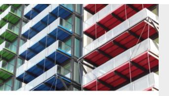
Designed by ROGER STIRK HARBOUR AND PARTNERS the Merano residencies at the Albert Embankment London consists of 40 luxury apartments overlooking the Thames. MACALLOY BALCONY HANGERS were used in various inclinations to support the balcony deck anchored into the structure using a "gallows" concept giving an Aesthetic feel and design. This solution maximises the floor area and gives a large viewing platform across the Thames.
