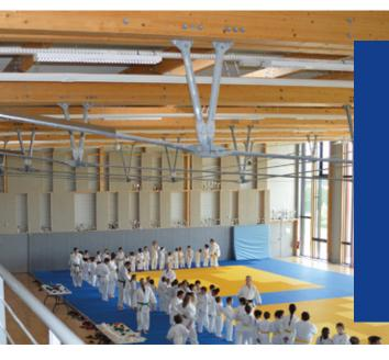
JUDO GYM, CHATEAUBRIAND. Macalloy 460 galvanised tie rods and fixed end compression struts form part of the main roof support system allowing the roof to span over 25 metres whilst maintaining a lightweight and aesthetically pleasing appearance. Macalloy SC460 stainless cables provide a discrete form of secondary bracing to the main structure. Macalloy 460 galvanised tie rods were also used to provide attractive and discrete vertical cross bracing support to the building façades.
